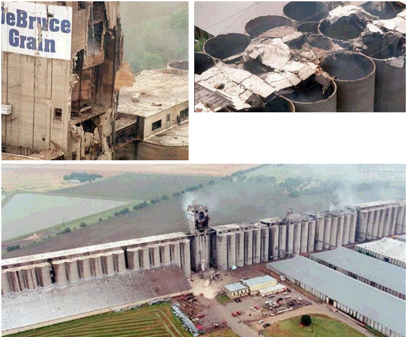
Figure 1: These pictures demonstrate the destructive potential of dust explosions. Note that explosion propagated through the facility with multiple secondary explosions. This facility processed and stored grain. Seven employees were killed in the explosion (Grose, 1998).
